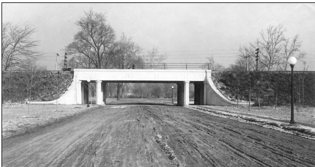
Figure III.14 The subway provided vehicular and pedestrian access through the railroad embankment. (R-LP0008_13260_subway.jpg IHS)
