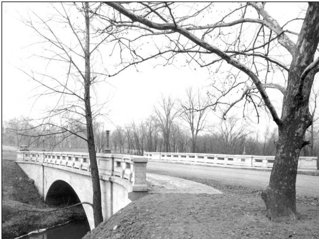
Figure III.12 View of the reinforced concrete Pagoda Drive bridge built in 1923, with open turf slopes and two trees; the larger one is a native sycamore. (R-8_sbridge.jpg IHPC)
